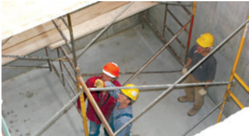
Hard hat area in the construction zone.
