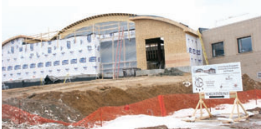
A view of the west side of the museum under construction.
